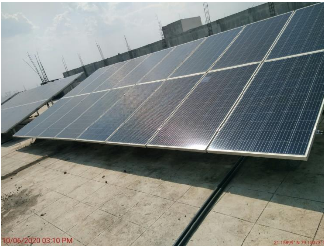
Meter, Inverter and Solar panel of Solar Power plant of capacity 50kW on the Roof of Taywade College
